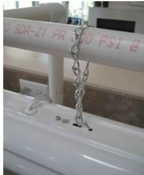
Figure 3 Detail of chain and "S" hook attachment
