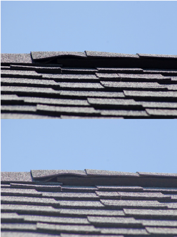
Figure 8. The dark spot is a suspected entry point for bats. In figure 9 light is reflecting off a board showing that entry is blocked. Photos by Stephen M. Vantassel.
