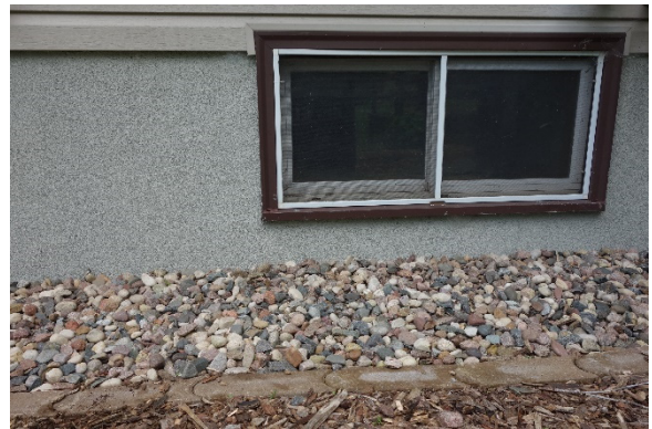
Figure 1. Stone or crushed rock can modify habitat around a building to reduce the availability of food, water, shelter, and access. Photo by Jan Hygnstrom.
