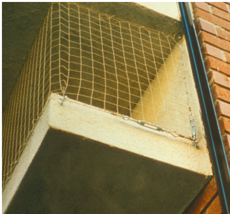
Figure 5. Nets are used to prevent birds from accessing a porch. Photo by Unknown.
