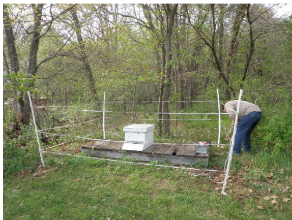
Figure 6. Installation of a polytape fence to protect a beehive. Photo by Jan Hygnstrom.
