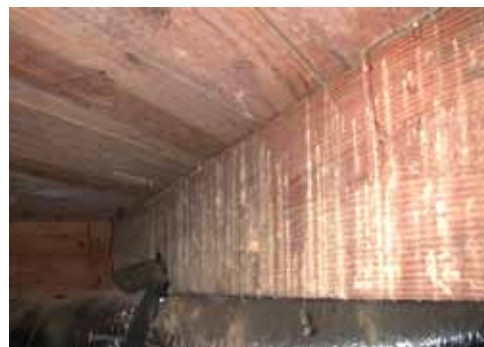
Visual evidence (frass streaming from exit holes) of an active anobiid powderpost beetle infestation in a crawlspace joist.
