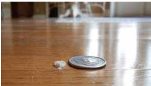
Frass from a true powderpost beetle emerging from hardwood flooring.
