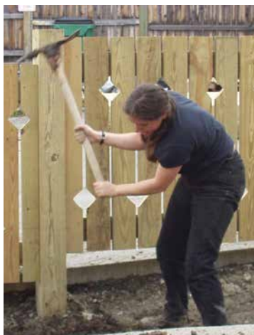
Using a pickaxe to break up compacted soil on a former parking lot site.
