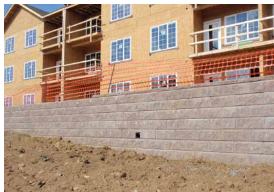
A retaining wall with drainage pipes is a practical solution for a very steep slope.
